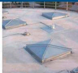
Roof explosion vents
