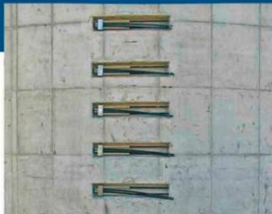
Anchor pockets for post-tension tanks
