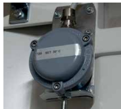
Termostato ambiente Ambient thermostat
