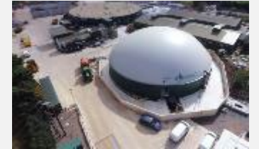
Gorst Energy (Clyst St Mary, outskirts of Exeter)
