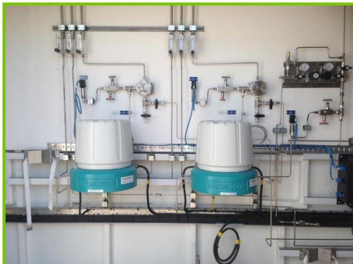
*Elster Gas Chromatographs for Biomethane CV, Ofgem C6+ analysis and GS(M)R compliance*
