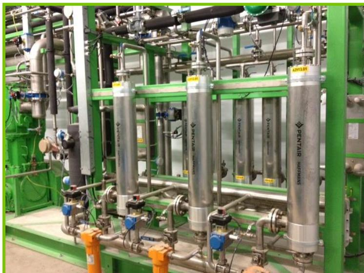
*Membranes used to separate the CO<sub>2</sub> from the CH<sub>4</sub>*
