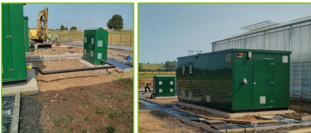
*Elster Grid Entry Unit and Remotely Operated Valve packages*
